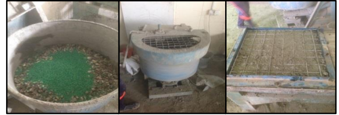
Figs.3. preparation of concrete slab
