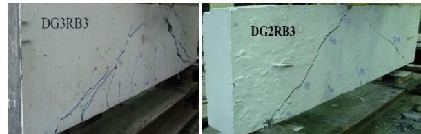
Figure 10: Crack pattern for directly loaded beams
