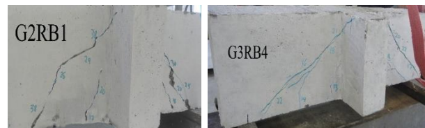
Figure 9: Crack pattern for indirectly loaded beams
