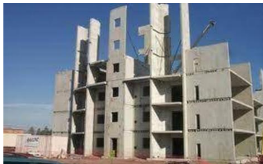
Figure 3. Illustrative photos of creating a prefabricated building
