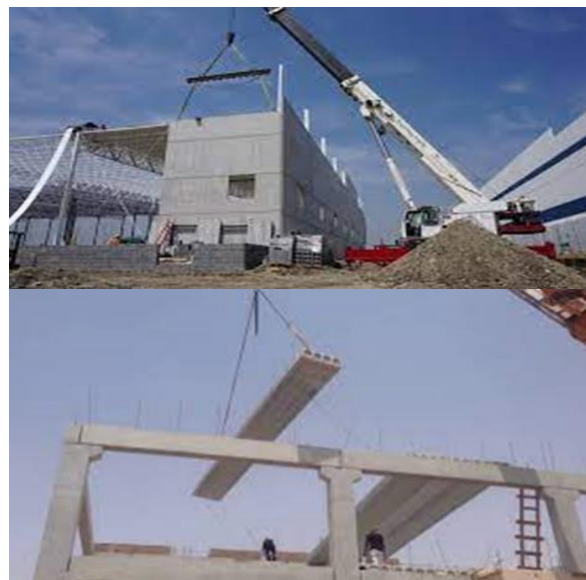
Figure 4. Illustrative photos of creating a prefabricated building
