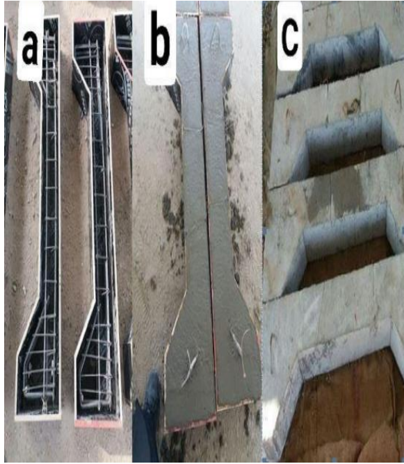
Figure 3. Phases of the casting process
