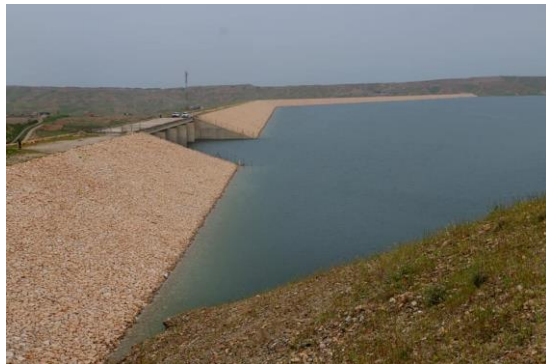
Figure 1. Khassa Chai dam
